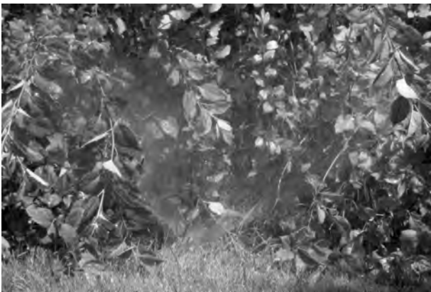
Figure 8-12 Shrub bed irrigation is complicated by growth of plants in the bed. In this case, shrub foliage has distorted the spray pattern, rendering this head ineffective.
