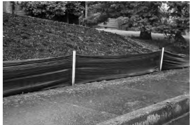
Figure 3-2 An erosion control fence can be an effective way to minimize on-site and off-site erosion during construction.
