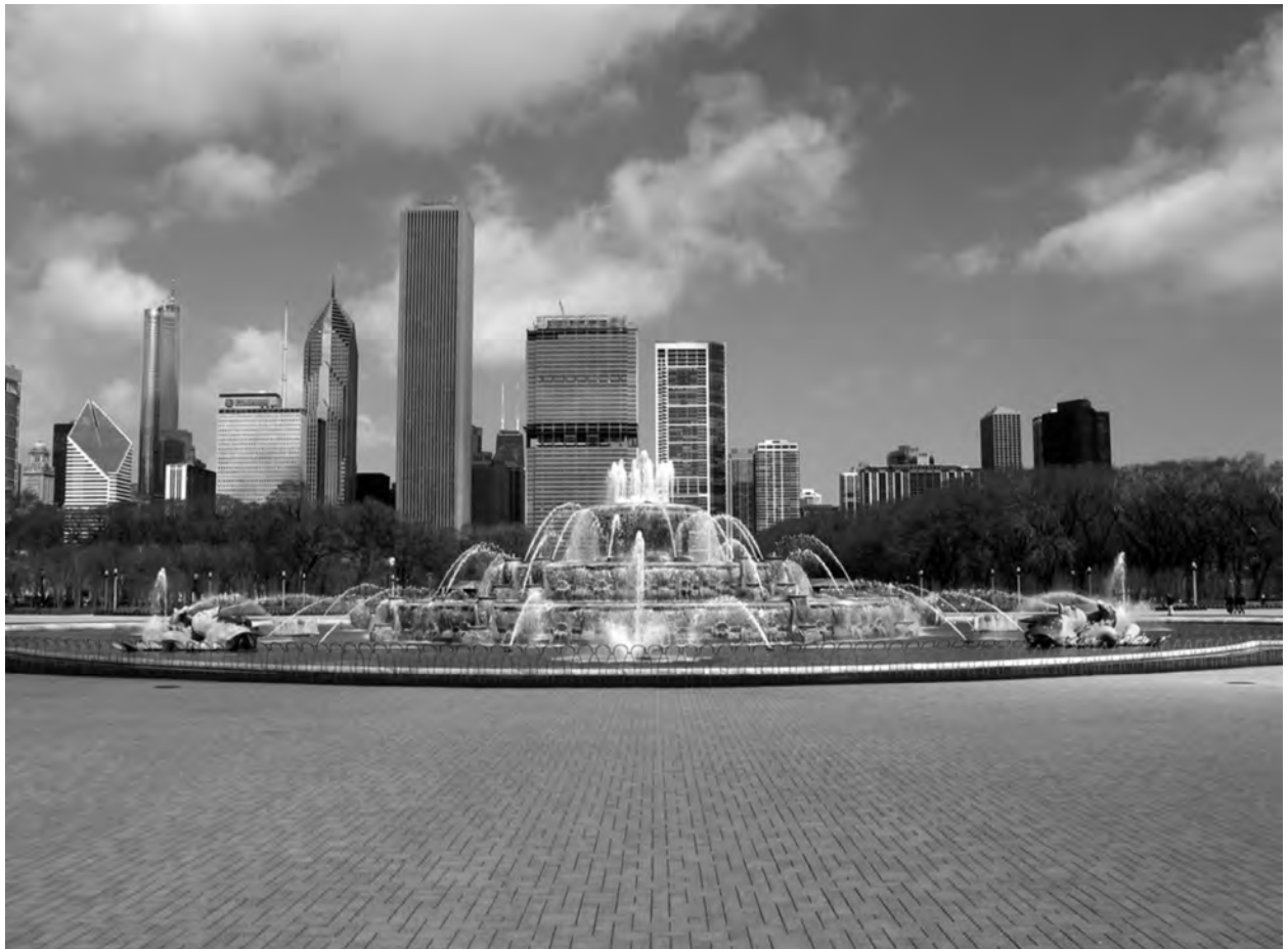
Figure 3-16 This public fountain in Chicago, Illinois, was surrounded with permeable interlocking concrete pavers. The result is a beautiful outdoor space and a large hardscape area that does not have runoff. Courtesy of Unilock, Inc.
