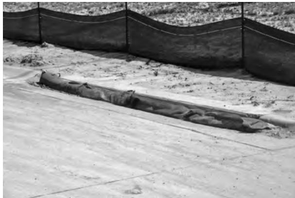
Figure 3-7 The soil erosion that has occurred on this construction site has ended up in the street and adjacent to the curbs. It will be hard to avoid polluting the storm sewers as this site is cleaned up.
