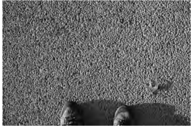
Figure 3-17 Pervious concrete is a sustainable hardscape alternative. The large pores allow water to quickly flow through the paving material to the base below.
