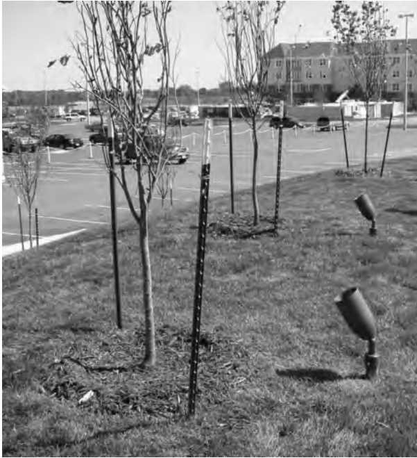
Figure 4-14 Uplighting is an effective way to highlight certain plants, but the location of these lights in lawn areas makes maintenance difficult and time consuming.
