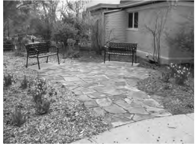
Figure 3-14 Limestone salvaged from a demolished retaining wall was used to create a functional patio for this seating area.
