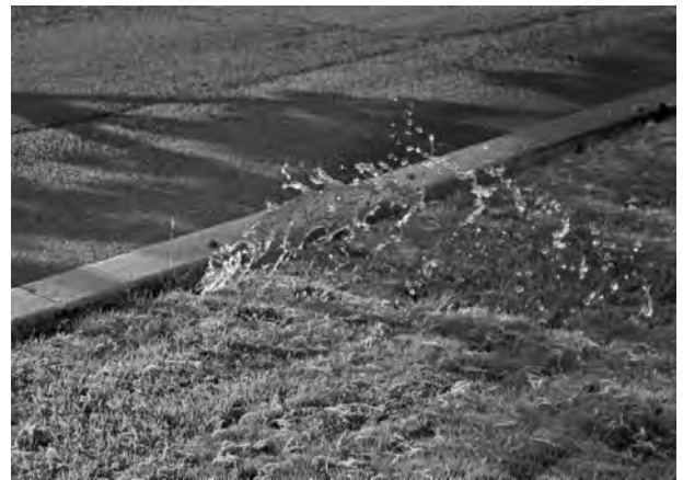
Figure 9-8 Broken heads may go unnoticed until parts of the lawn start to turn brown from drought.
