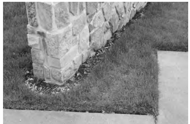
Figure 4-6 This maintenance problem is easily fixed by enlarging the unmowed area adjacent to the wall.
