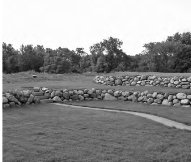
Figure 3-8 Boulders that were uncovered during excavation on this site were used to create a series of retaining walls.
