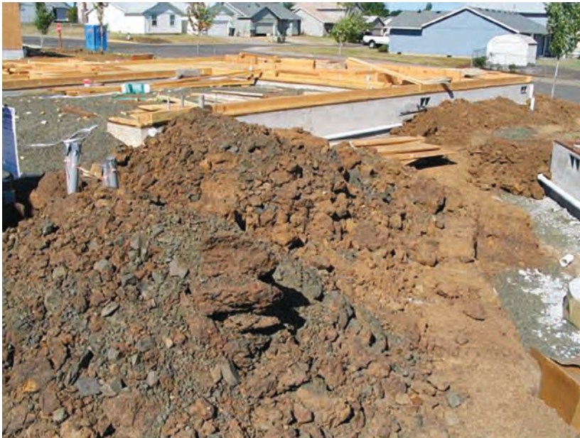
Color Plate 3-1 Poor-quality subsoil often ends up layered over the original topsoil, creating a poor rooting medium for newly installed plants. Courtesy Neil Bell.
