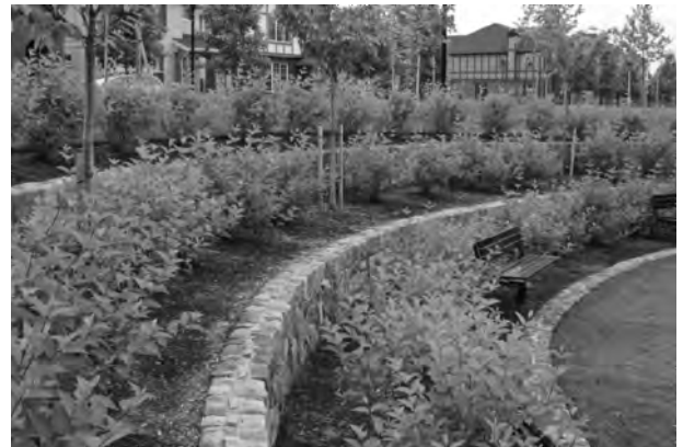
Figure 2-17 Short retaining walls were used to create level terraces for plantings in this design. The series of terraces gives the site an enclosed feeling and reduces noise from a nearby road.
