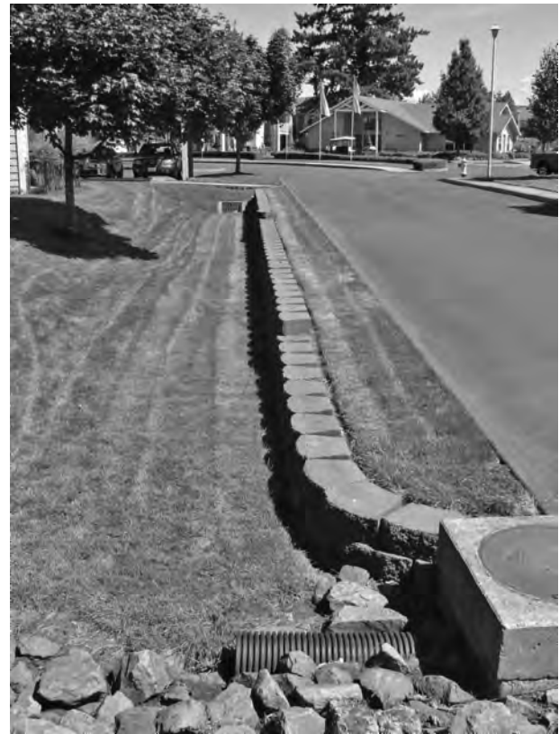
Figure 4-22 The concept for this bioswale is good. However, the block retaining wall makes it difficult to maintain. A better alternative is to remove the wall and plant the area with species that can handle periodic flooding.
