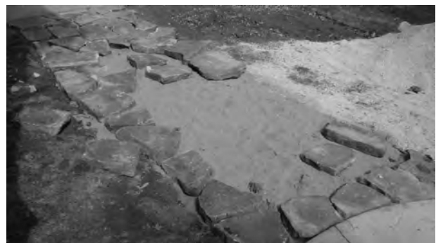
Figure 2-19 Limestone salvaged from a retaining wall demolition project was recycled to create this walkway.
