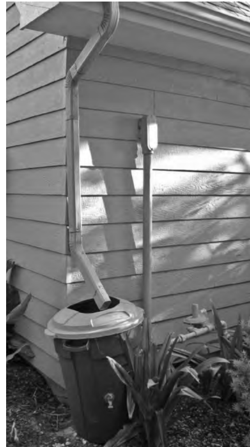
Figure 4-20 A rain barrel attached to a downspout is an effective way to capture rainwater so it can be used for irrigation. This concept is applicable to commercial buildings and landscapes as well.
