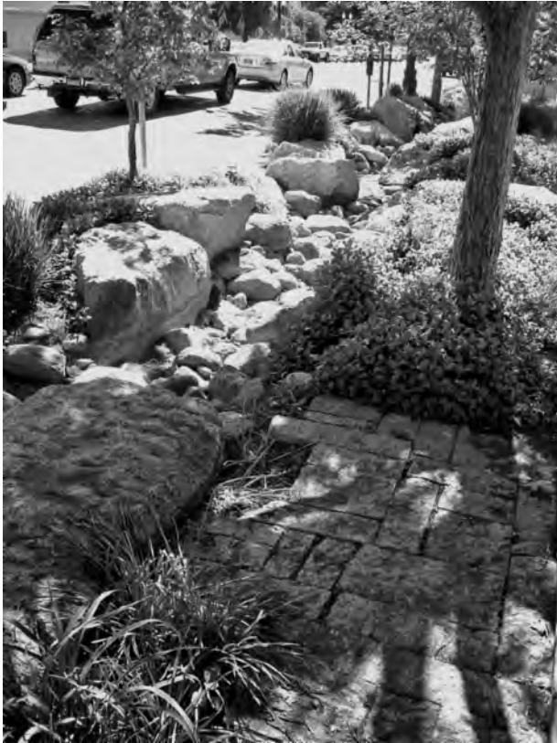
Figure 2-18 The dry river bed installed adjacent to this street serves as a collection point during heavy rainfall events and prevents storm water runoff from reaching the storm sewer.
