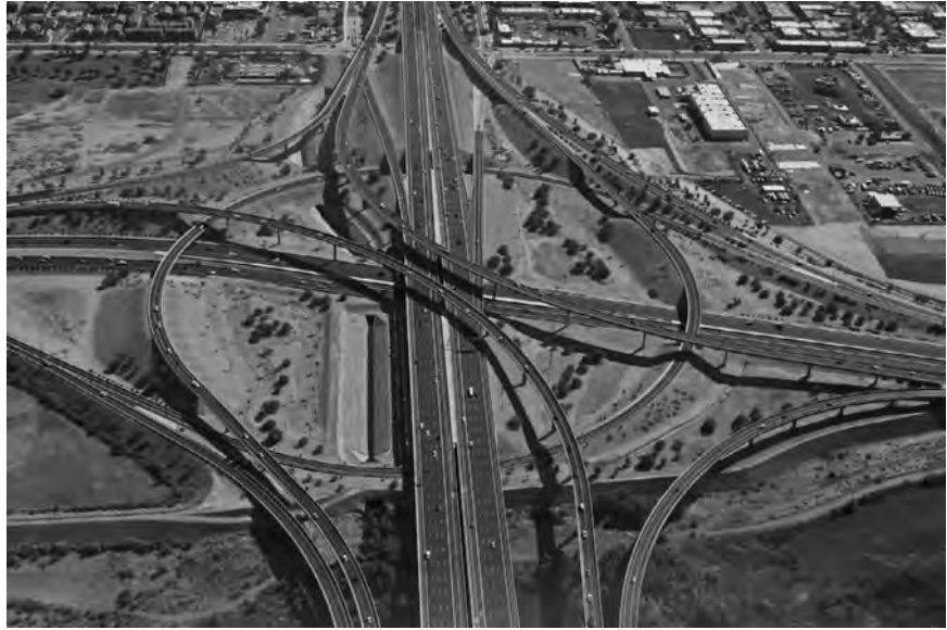
Figure 1-5 This freeway interchange demonstrates our ability to impose our will on the land. Ian McHarg believed it was possible to design the built environment in harmony with the natural environment and avoid the problems associated with thoughtless development.
