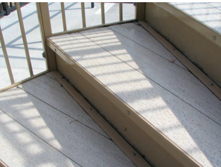
Color Plate 3-3 A composite wood material was used to build these steps. The product looks like wood but has a longer life span and requires less maintenance than wood.
