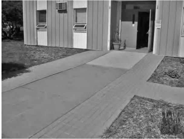
Figure 2-20 The entrance to this building was widened to improve access by adding concrete pavers to the edges of the existing walkway.
