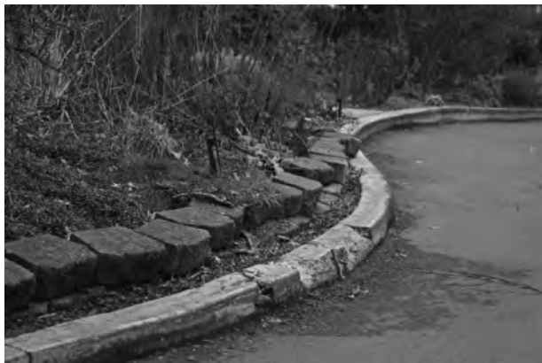
Figure 2-10 This narrow driveway between two buildings does not provide adequate room for trucks. A single layer of wall block was installed to protect the plants and irrigation system, but it and the curb continue to be damaged by truck wheels.
