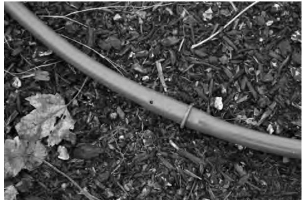
Figure 4-18 Low-volume drip irrigation systems are an effective way to irrigate planting beds.
