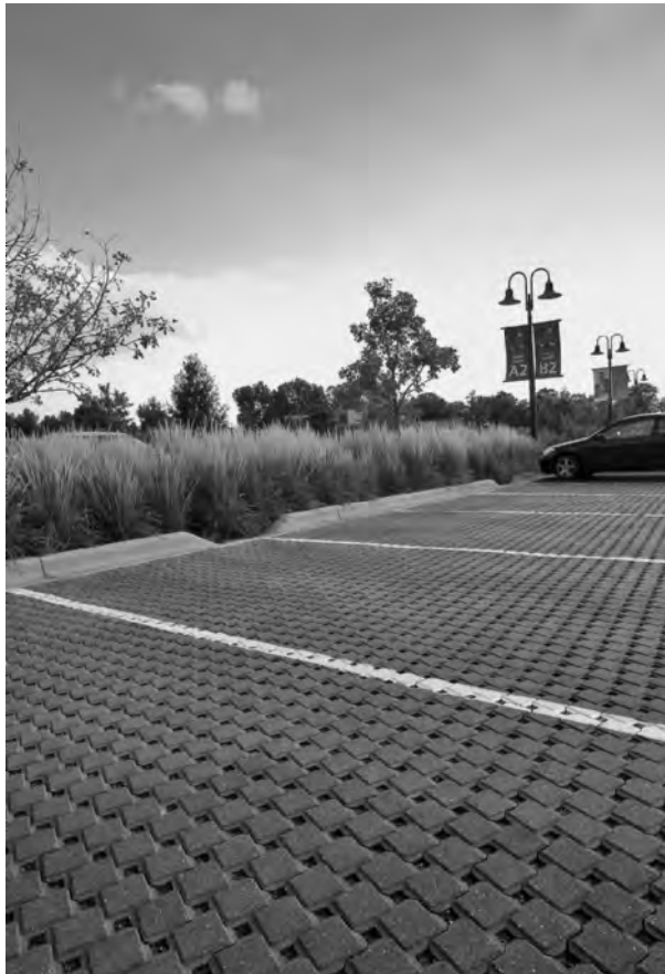
Figure 4-12 This parking lot area at Morton Arboretum was converted to permeable interlocking concrete pavement to eliminate storm water runoff.
