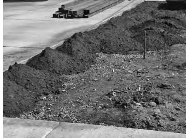
Figure 3-6 Topsoil (the dark soil in this image) has a much different composition from subgrade soil and should be tilled into the existing site soil to prevent a soil interface problem.
