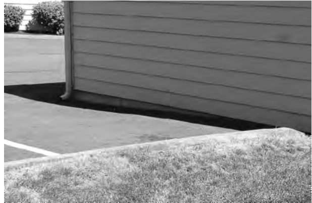
Figure 2-23 The downspouts on this commercial site empty directly onto a hard surface and contribute to the site's storm water runoff.
