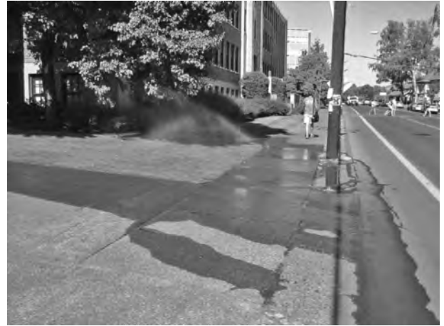
Figure 9-7 Poorly adjusted sprinklers often result in wasted water, as noted here, where water is running down the street due to sprinkler overthrow.
